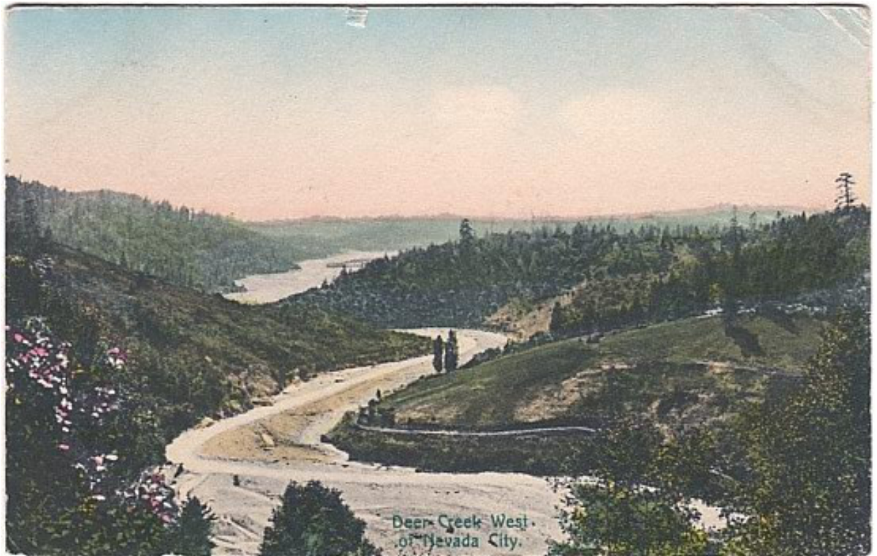
Deer Creek Circa 1908, looking west from immediately downstream of Champion Mine. Note how channel is completely filled with gravels from mining activities.
