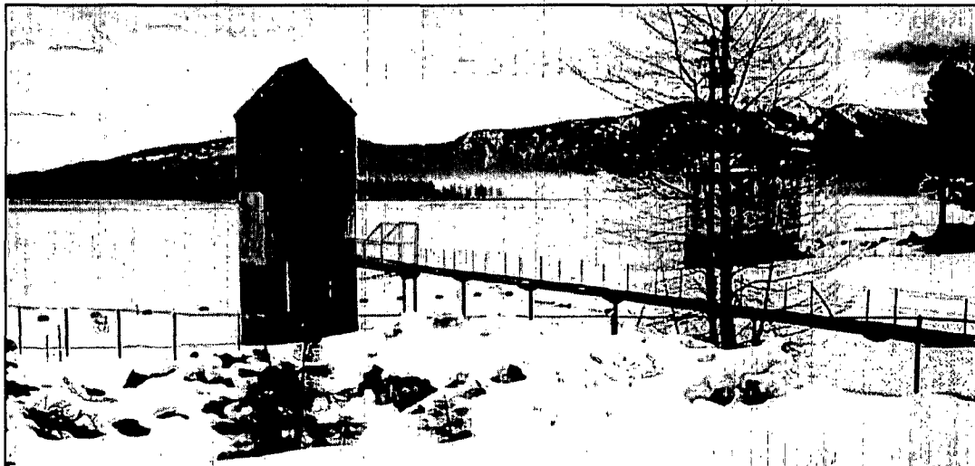
Figure 1-1. A view of Prattville Intake and Lake Almanor.
