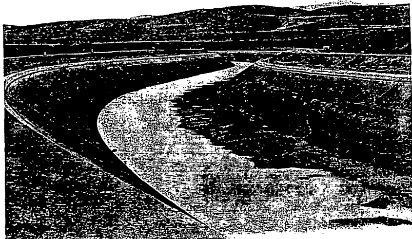
Figure 2. Typical sediment bar on the invert of the Delta-Mendota Canal as seen when it was dewatered.
