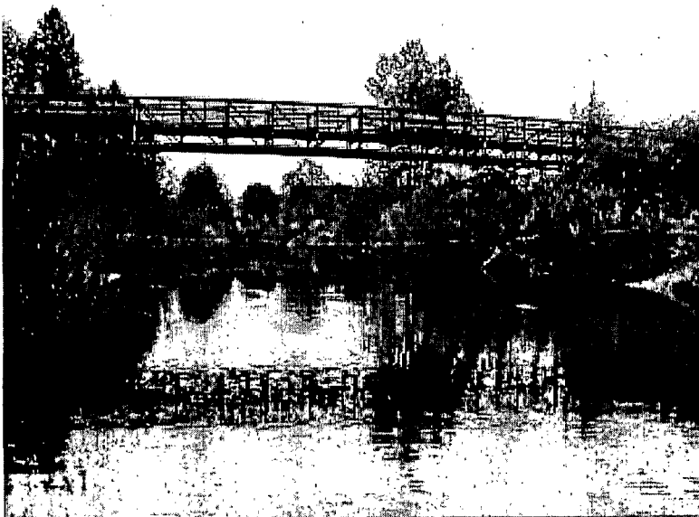
Figure 24. Spanish Creek at Hwy 70 (Gansner Park)
