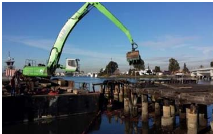
Photo 2b. Removal of the dilapidated pier at Union Point Park, Oakland, across from Coast Guard Island.
