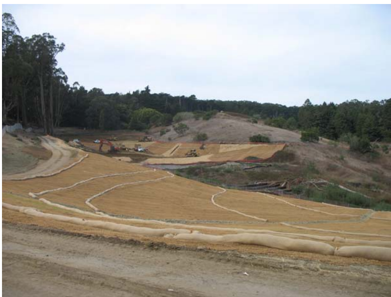
Example of the use of fiber rolls, mulching, silt fencing and sediment controls installed after cleanup at a former landfill at the Presidio of San Francisco.
