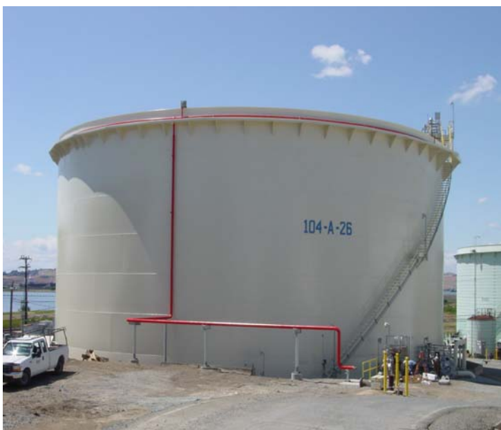
Photo 2: New Double Bottom Tank with Leak Detection
